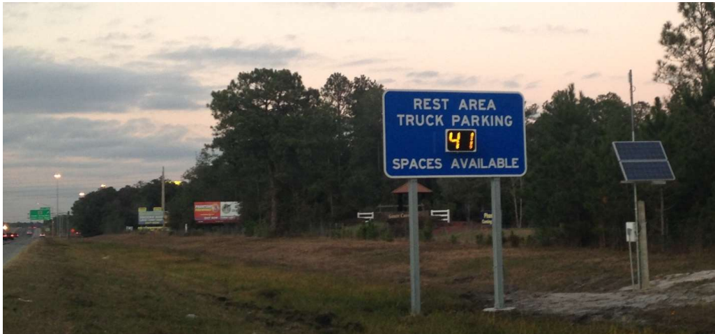
Pilot TPAS Sign on I-95 in St. Johns County
